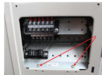
Terminal Board Screws
